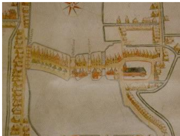
De Dam in 1648
